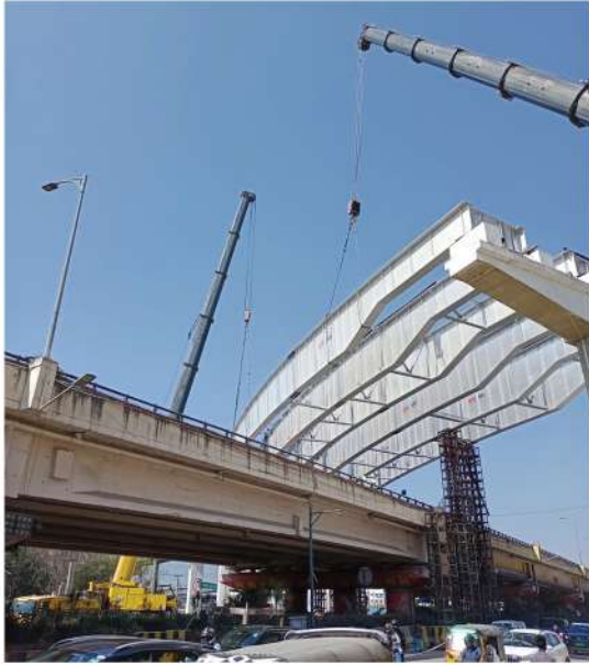
64-METER SPAN FLYOVER
