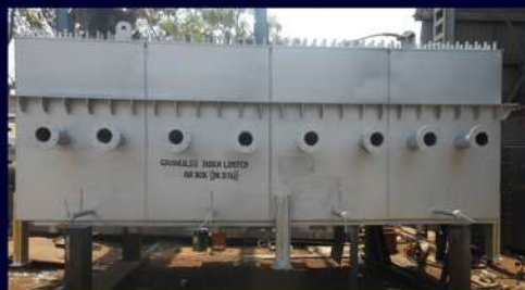
AIR BOX WITH S.S PIPE TO M.S PIPE WELDING ON TOP TO GRANULES INDIA LTD.
